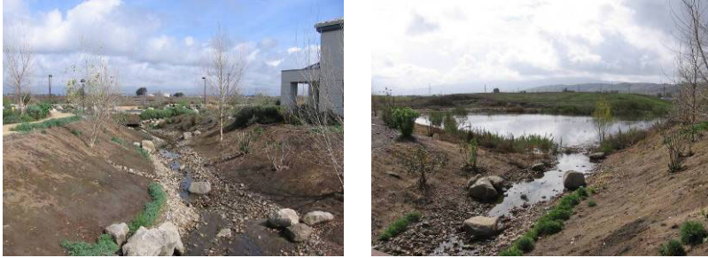
Figure 7: Channel and Detention Basin
