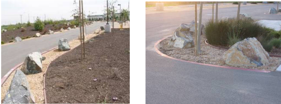
Figure 5: No curb and gutter
